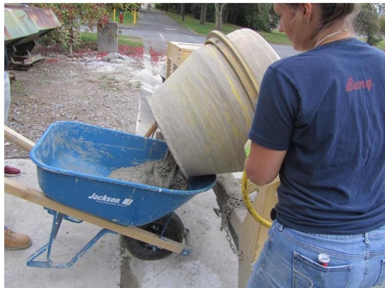
Figure 4-3: Removal of Concrete from the Machine Mixer in Preparation for Testing and Casting
